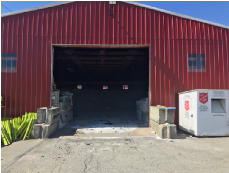
Salt Pile Storage
